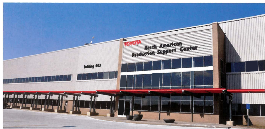
Toyota's North American Production Support Center training facility in Georgetown, Ky., serves Toyota plants in the United States, Canada and Mexico.
